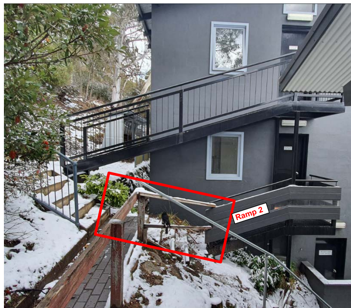
Install Barrier to comply to BCA clause D2.16.
